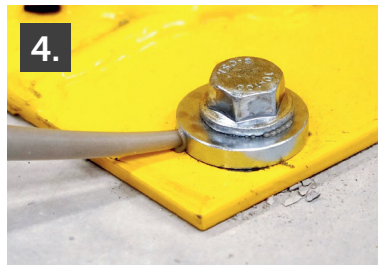
4.) Fill the annular gap between Concrete screw and fixture through the hole of the Filling Washer until resin leaks out of this hole.
