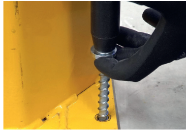
2.) Drive in concrete screw with filling washer until the anchorage depth h_{nom} is reached
